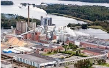
Paper mill: Fans, Compressors, Pumps, Electric boilers
