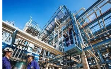
Process industry: Electrolysis, Fans, Pumps, Heating
